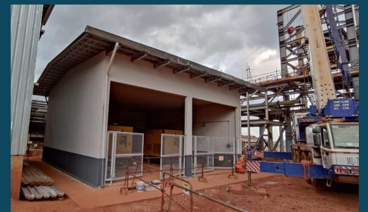
Obra Industrial - VALE S/A - MG
